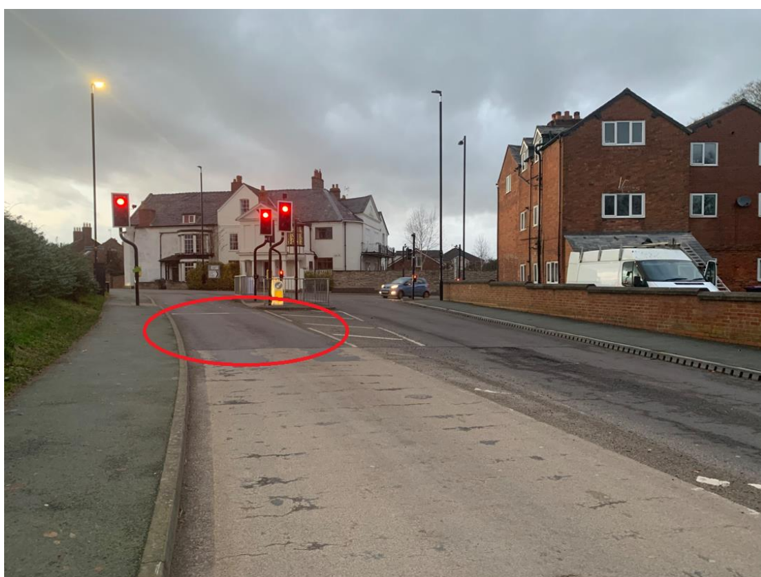
Looking north along Canal Way towards the signalised junction with the A495. The existing high friction surfacing does not extend to the stop line (circled) following previous surfacing
