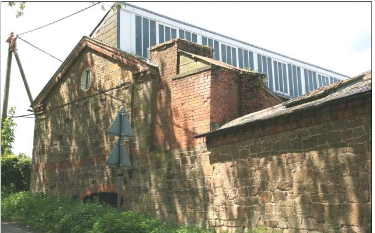
20. View from Birch Road, showing gable pediment, long dormer and brick steam engine bay
