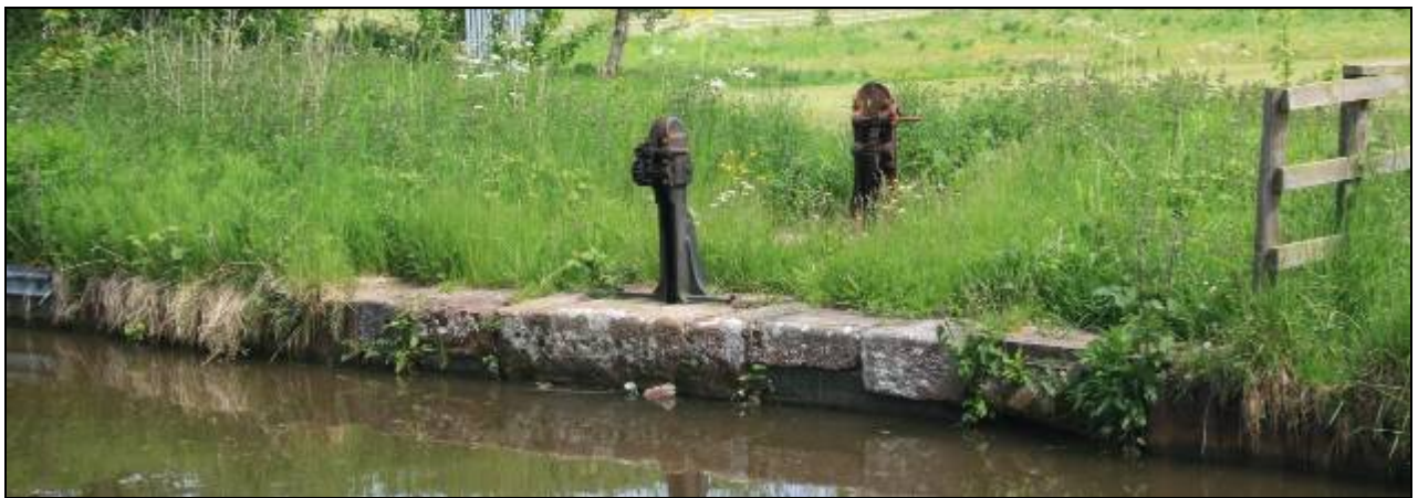
25. Gearing probably associated with the former boat house and dock
