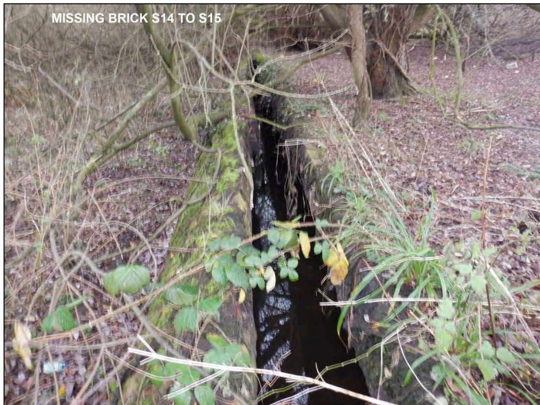
Figure 4.1: Open Top Culvert near Dairy Grove and the Cricket Ground
